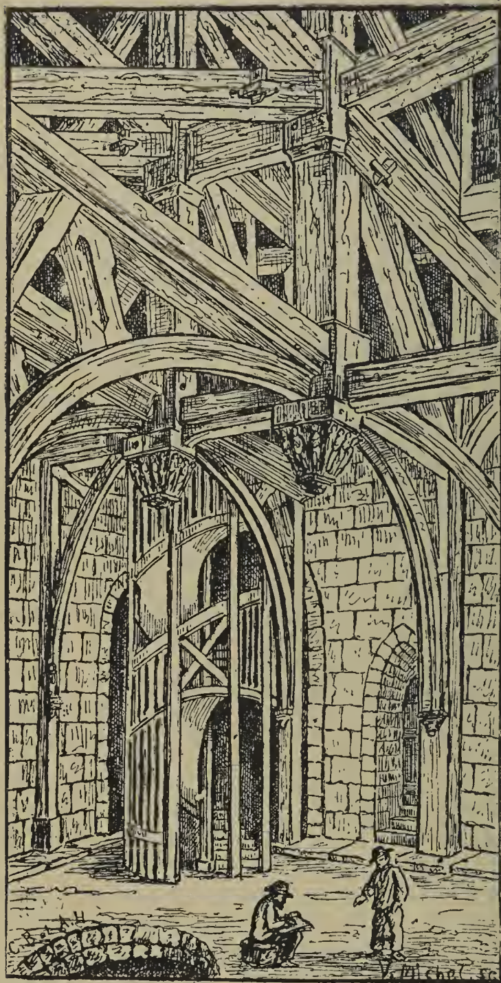
S.-W. BELFRY. TIMBER-WORK DESTROYED IN THE FIRE OF 1836.
